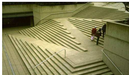
An example of steps incorporating a slope
